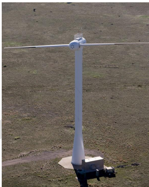
Figure 1: CART2 wind turbine at the NWTC with black CVG tape shown on the leading edge of the blades. Photo by Lee Jay Fingersh, NREL.
